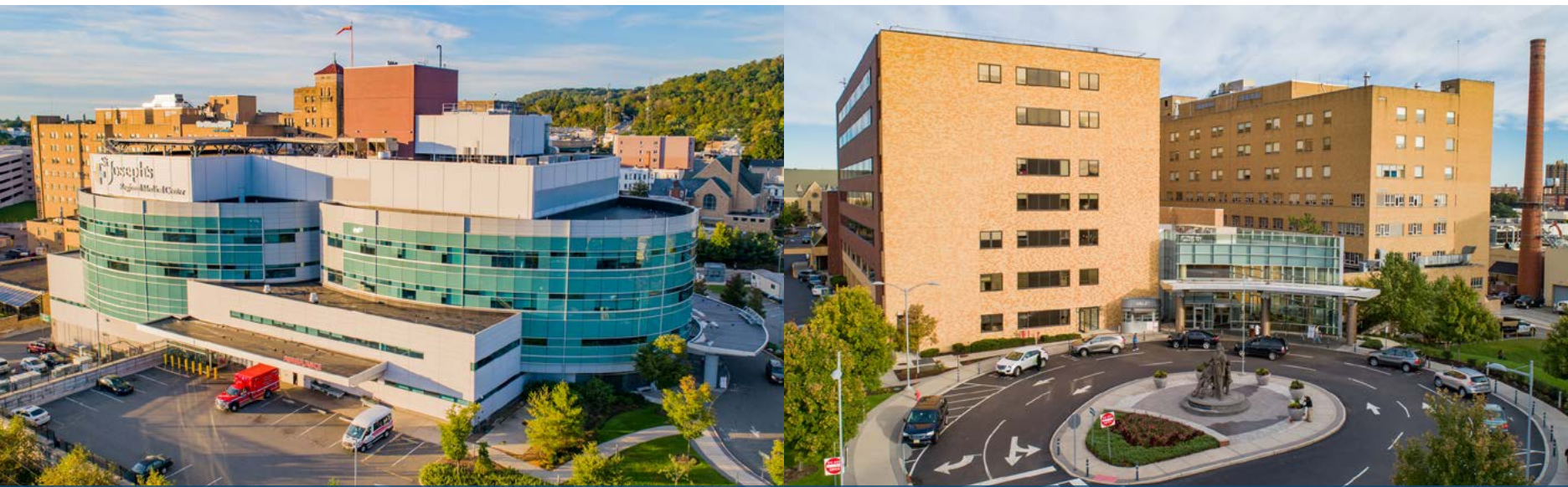
An exterior view of the Critical Care Building and helipad at St. Joseph's University Medical Center.
